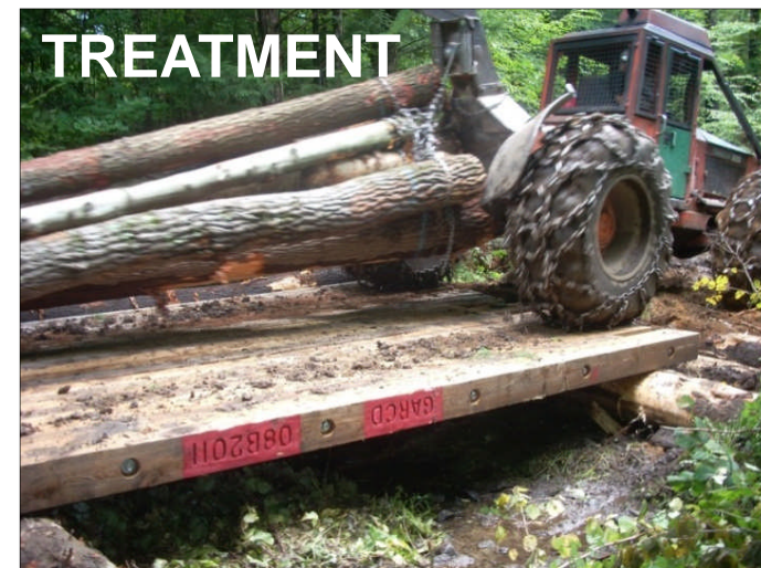
Temporary skidder bridge
