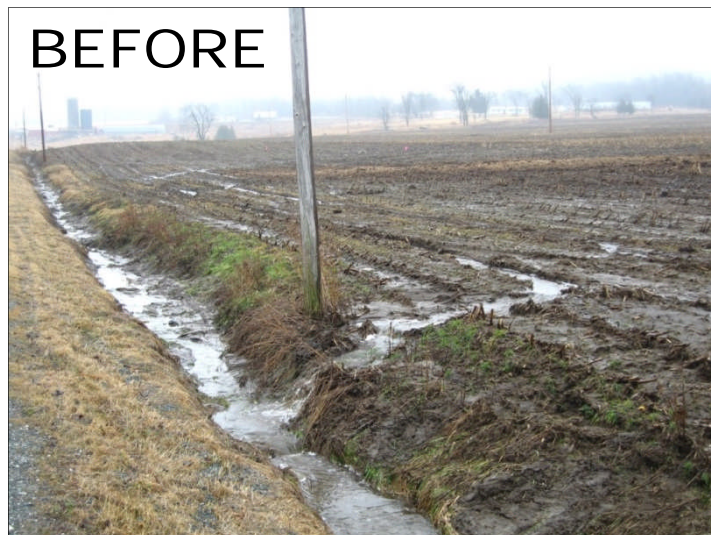
Runoff draining into ditch
