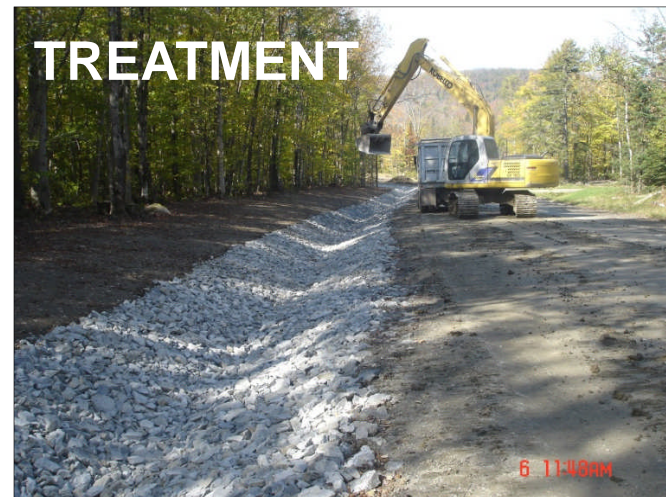
Ditch stabilization saves road and reduces erosion 12
