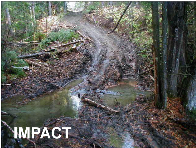
Unmanaged stream crossing at logging site
