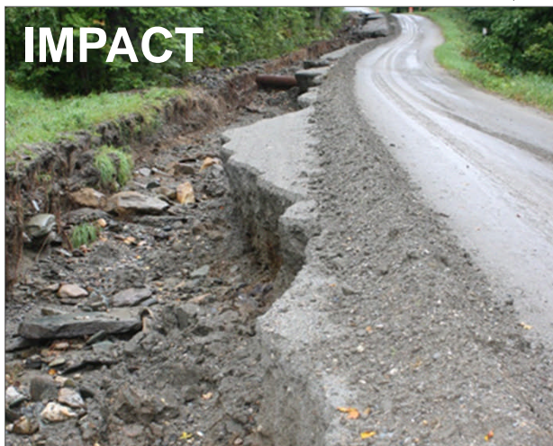
Eroding roadside ditch
